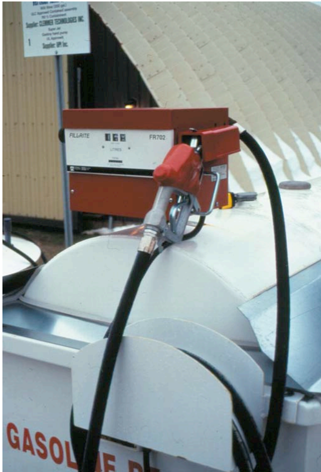
Figure 2. Fuel tanks can be placed in a dike to provide secondary containment in case of a spill.
